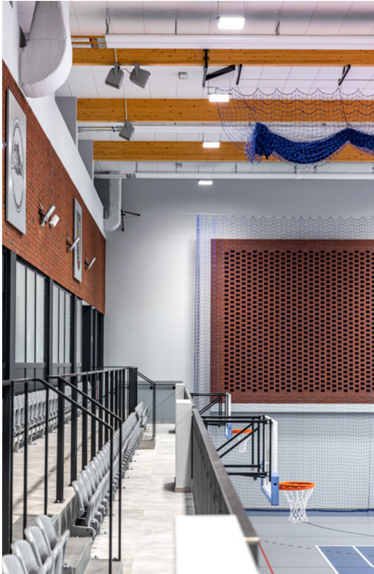
Lighting of the sports field in Gliwice
