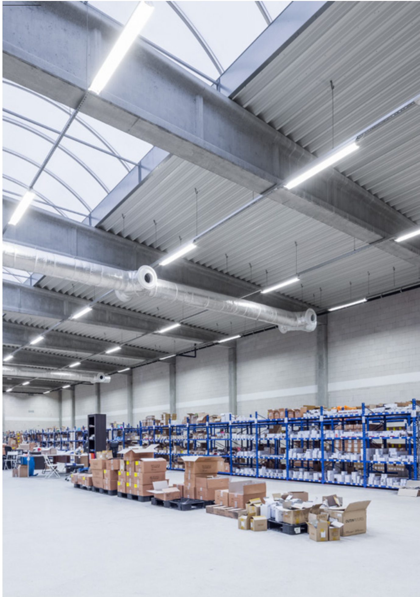
Application of Tores LED PC luminaires in a warehouse hall
